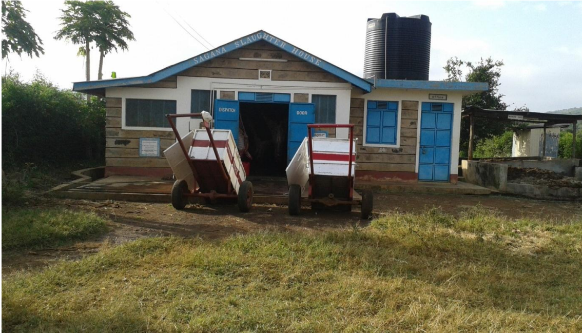
Sagana slaughterhouse building
