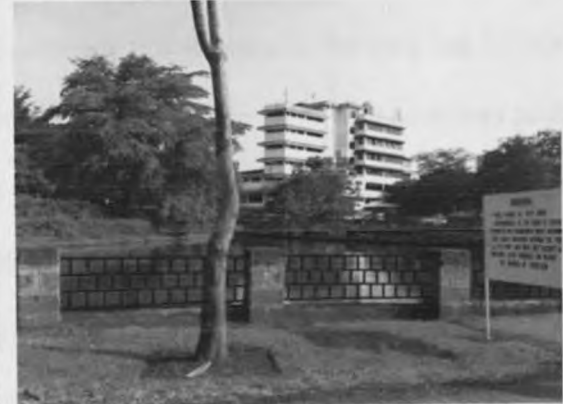
Plate 4.46. Safety barrier around the pond
