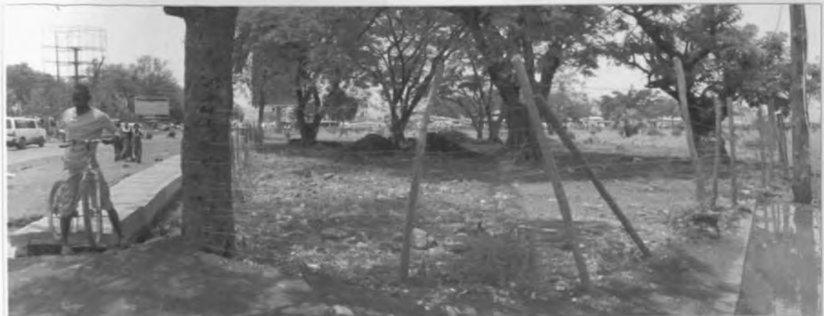
Plate 4.3. A view into Oile market park under restoration. Source: Author
