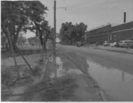
Plate 4.6. The neighboring road and buildings. Source: Author
