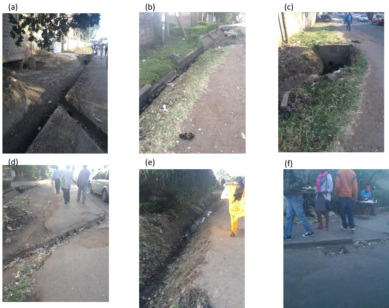
Figure 25: Existing conditions of storm water drainage infrastructure in South C.
