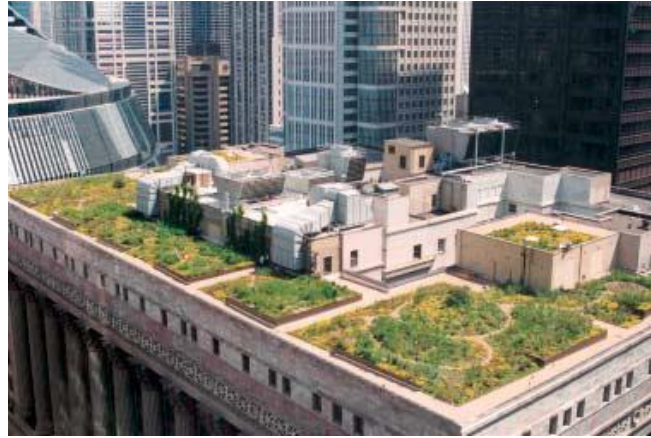
Figure 8: Green roofs to reduce the volume of storm water runoff (Source: Chicago's Water Agenda, 2003)
