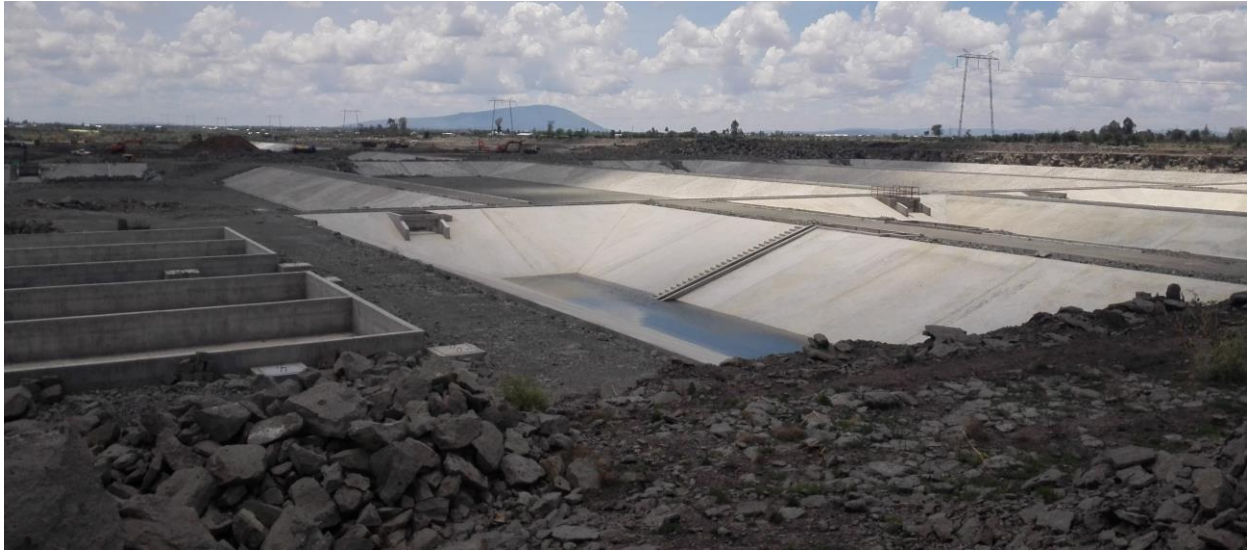
Plate 0:4: Section of the Ruiru Sewerage Works under Construction
