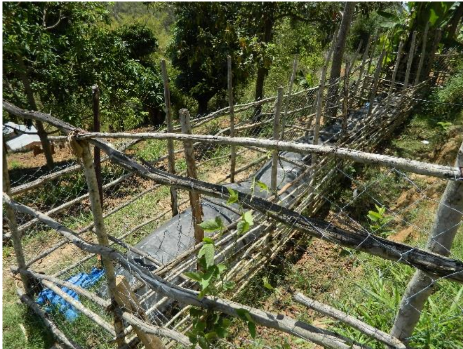
Plate 4.1: Plastic Digester is a biogas technology placed inside a trench with inlet and outlet pipes tied on both sides.it should slant at a slight angle for free flow of slurry. (Source: Field Data, 2014)
