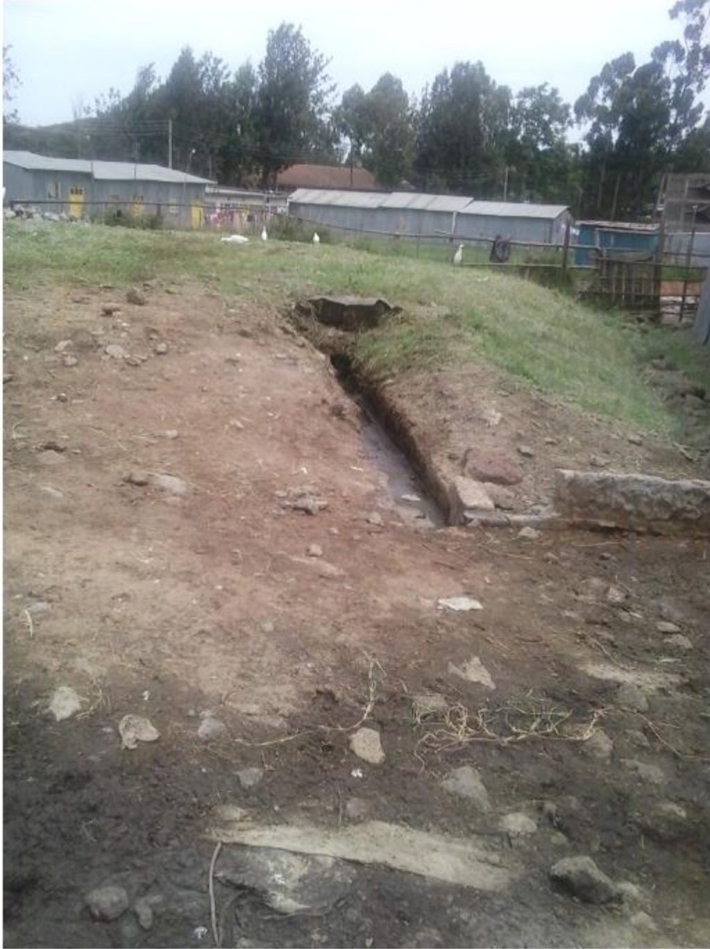
Fig. 1.3 Ongata Rongai Slaughter house first soak pit inlet point
