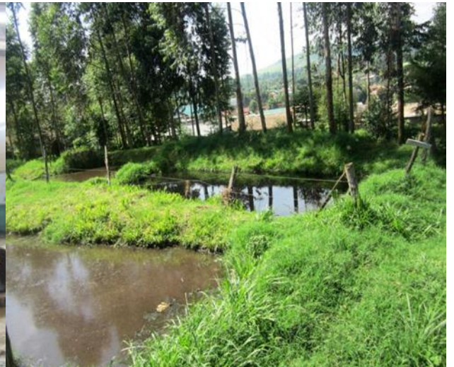
Plate 8.12: Lagoons for wastewater
