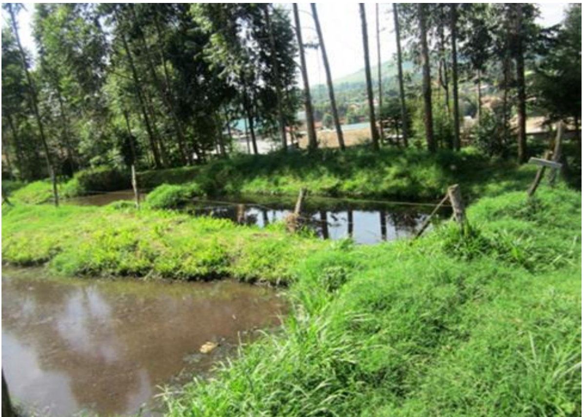
Plate 4.1: Lagoons for wastewater
