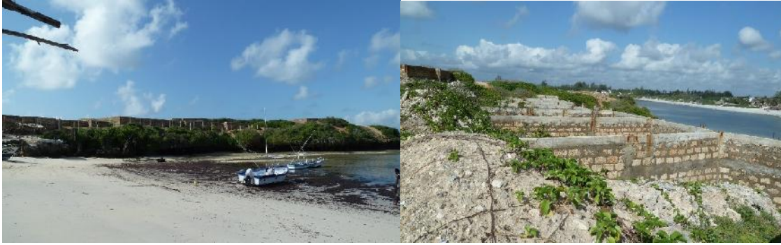
Figure 38: Illegal development on Blue lagoon headland
