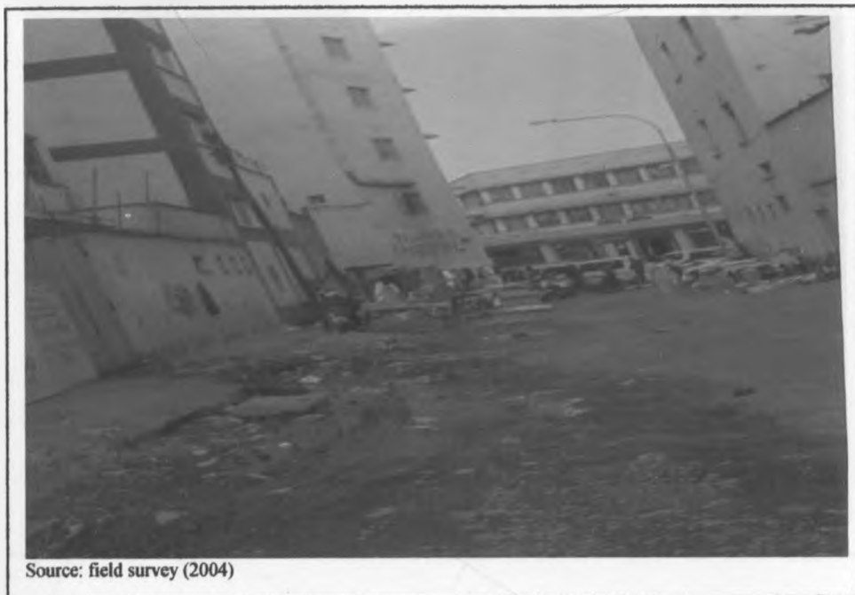
Plate 4.2. Waste Water Flowing Along Fire Station Lane
