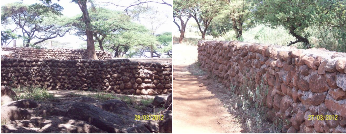
Figure 10: Protective perimeter walls within Tikondo spring.
