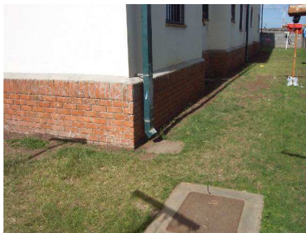
Plate 21: Sewage system at the backside
