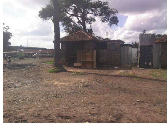
Plate 54. Buildings in disrepair
