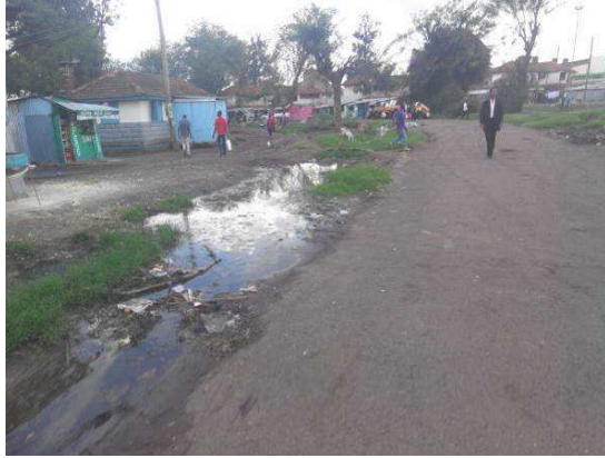
Plate 53. Clogged drainage
