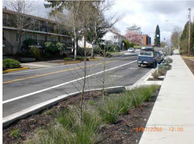
Bioretention Planter-Source: A. Omlid.
