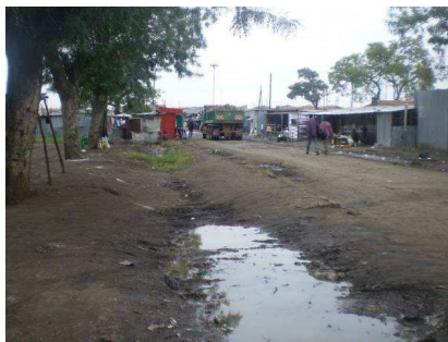
Plate 51. Poor state of roads
