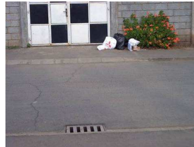
Plate 20: Subsurface stormwater drainage
