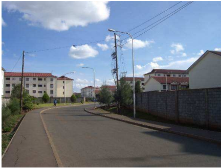
Plate 23: Street Lighting along circulation spine
