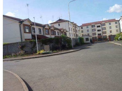
Plate 18: Redundant spaces not appropriate
