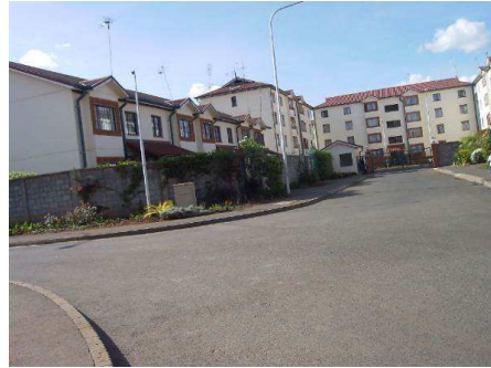
Plate 24: Street lighting for security
