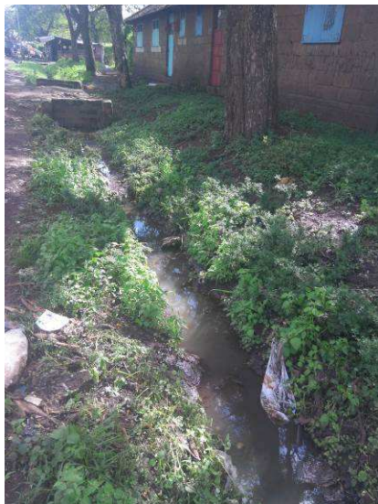
Plate 62. Stormwater in clogged drainage
