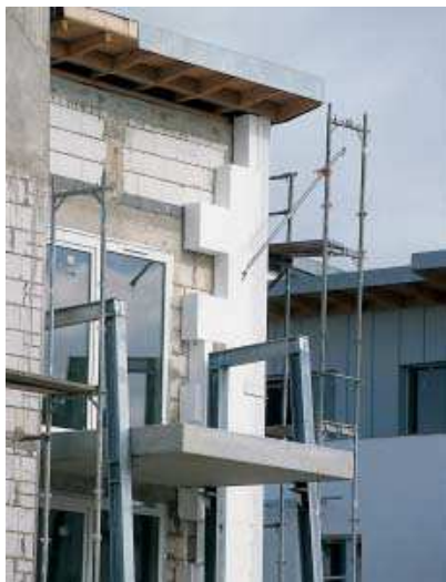
Plate 36. Wall insulation
