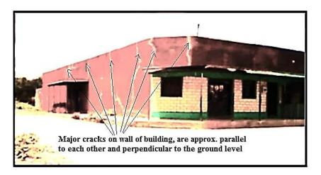
Plate 1.1: Photographic illustration of a cracks-infested prime building at Mutito-Andoa market centre in Mui Basin, can be an indication of challenging subsurface geological conditions
