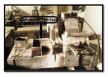
late 3.11: An electric-powered stone saw; showing mounted vise to the left-hand side
