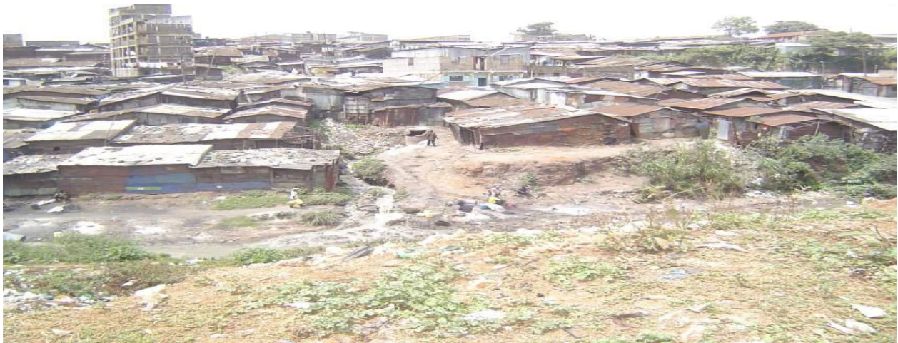
Plate 5.1 : Housing and drainage in Kosovo Village, Mathare Slum
