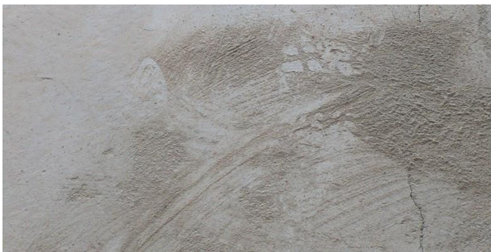
Plate 2.4: Dusting on Concrete Surfaces
