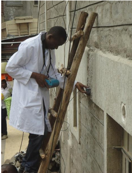
Figure 3.11: Undertaking structural tests using Profometer 5+ covermeter
