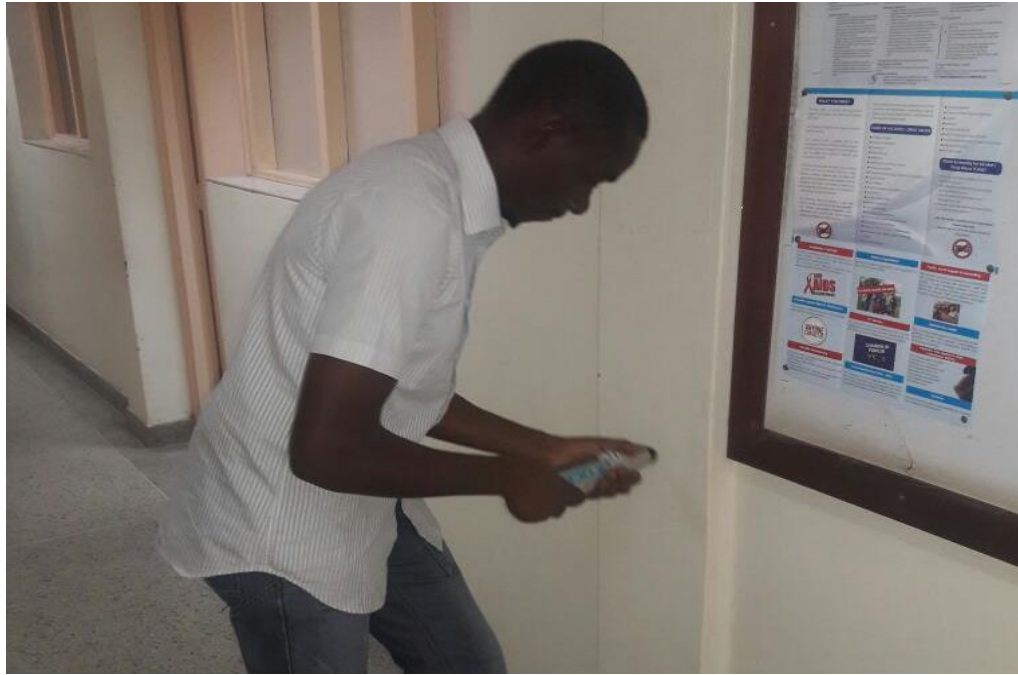
Figure 3.12: Undertaking surface hardness tests using Schmidt rebound hammer
