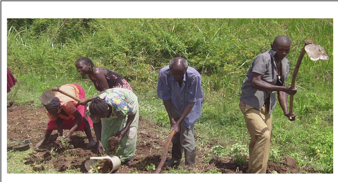
Figure 4.15: Community members digging trenches in Budalangi
