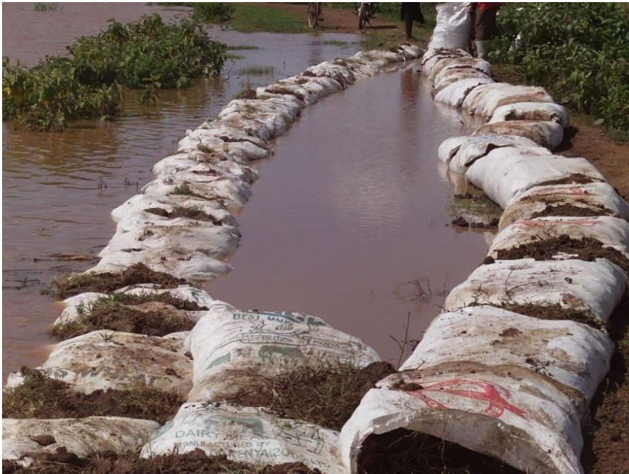
Figure 4.10: Sand bags in use to prevent floodwater in Budalangi
