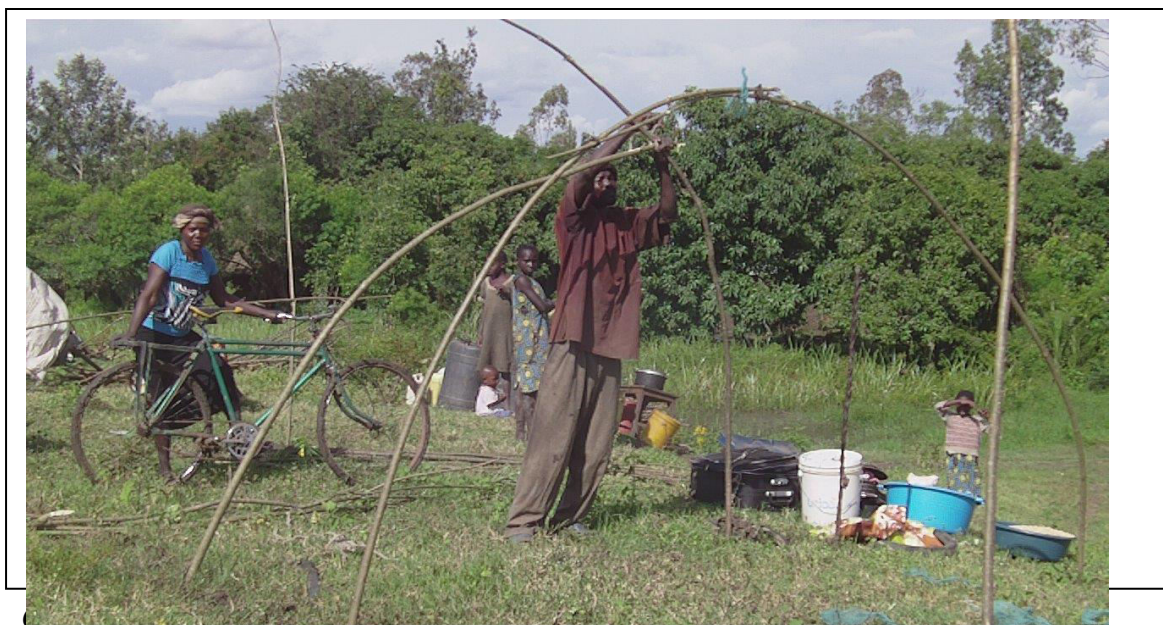
Figure 4.13: Community members in Budalangi constructing temporary shelter on safe ground
