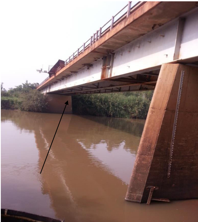
Figure 4.8: Measurement scale on Rwambwa Bridge on river Nzoia in Budalangi
