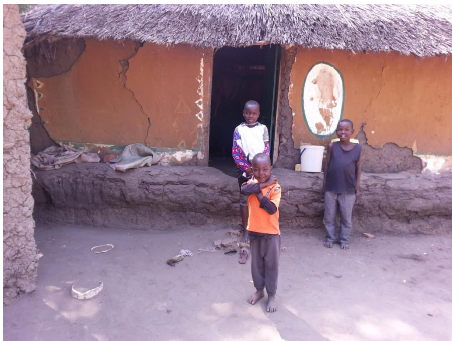
Figure 4.11: A house elevated from the ground in Rukala sub-location in Budalangi
