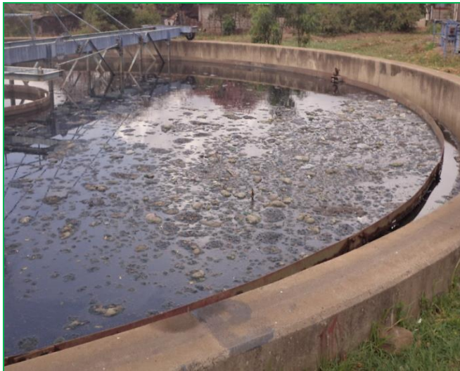
Figure 2.14: Decommissioned clarifier with water
