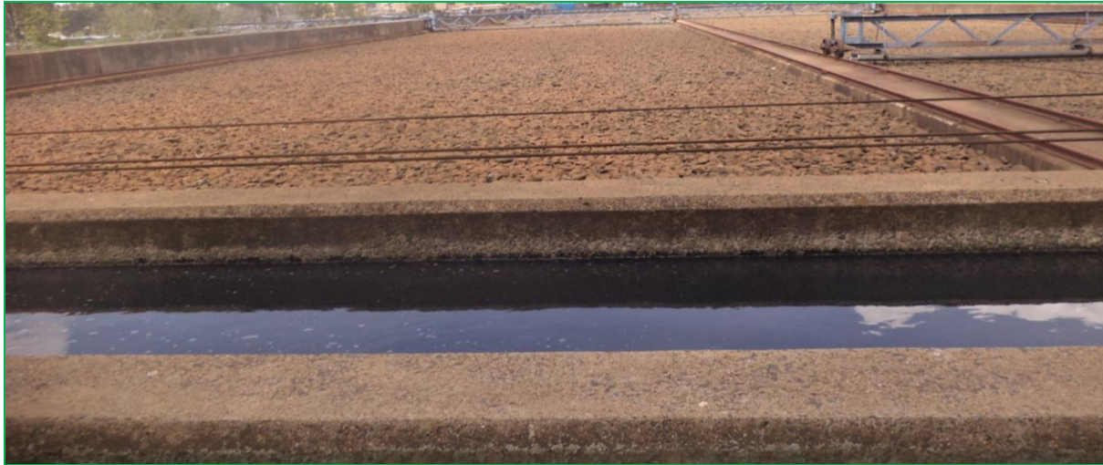
Figure 2.9: One of the filters at Kariobangi Treatment Works
