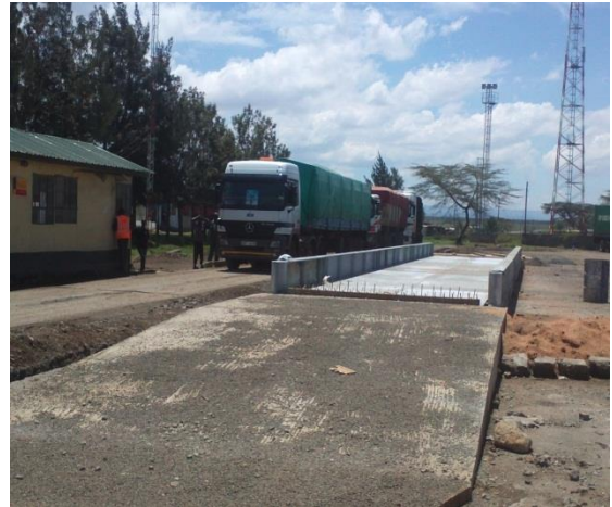
Plate 8: Adjacent single axle unit in use Source: Author (2014)
