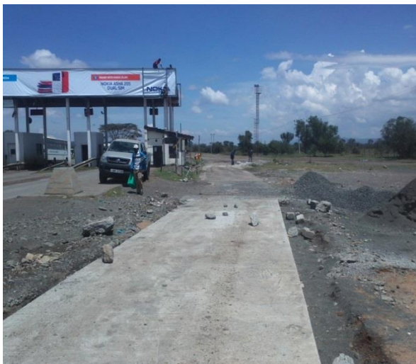
Plate 3: 2 nd weighbridge closed for repair at Gilgil
