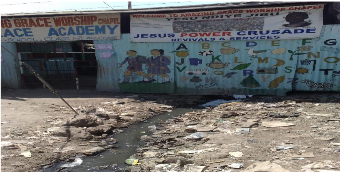
4 Sewage and Noise hazards: Exhibits sewage flowing through school and a worship place adjacent to it.
