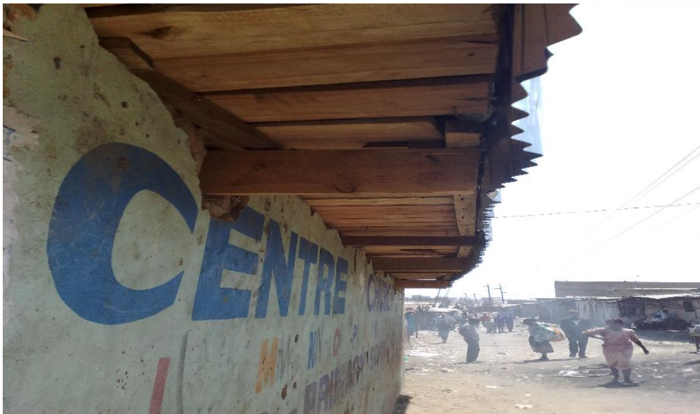
2 Photo of a classroom floor: Exhibiting gaping holes on the classroom floor base which pose a great health hazard to students
