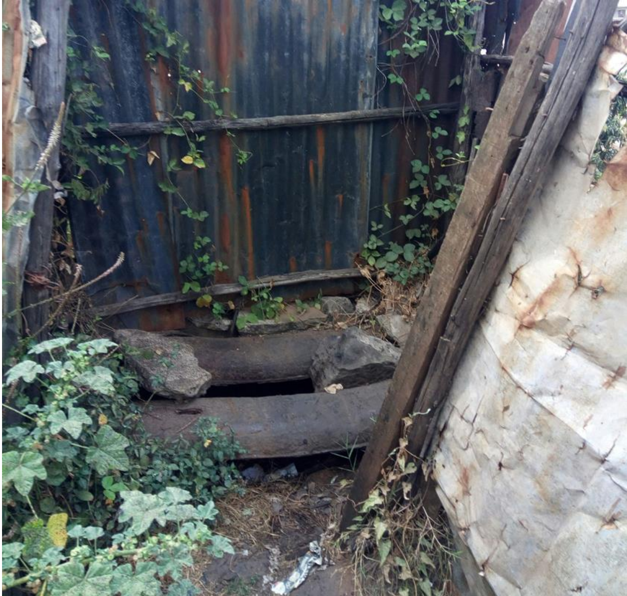
Figure 4. 6: Typical shallow household unimproved pit latrine with metal slab commonly found in the two study areas.
