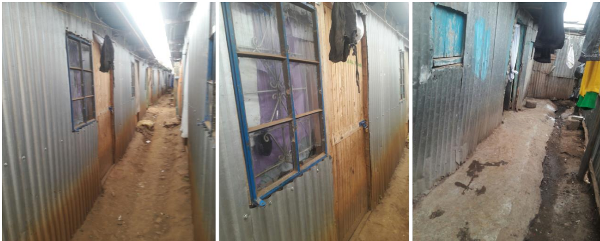
Figure 4. 2 Multi-family congested substandard buildings of ~ 115 rooms, made of corrugated iron sheet houses
