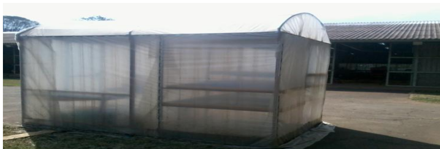
Figure 4.1. Polythene green house solar drier
