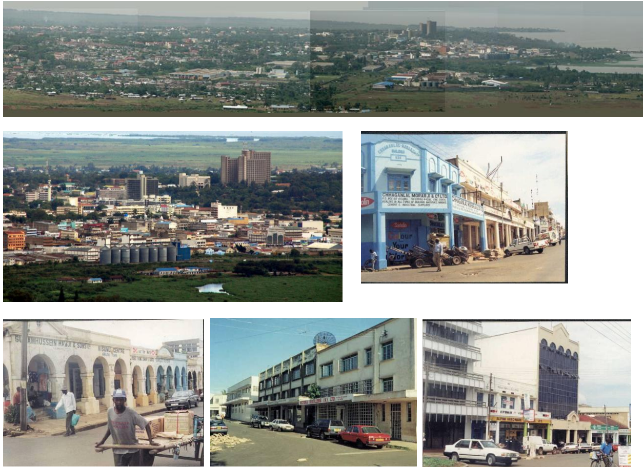
Fig. 5.28: The general skyline of Kisumu and the various building typologies and architecture. Source: Author
