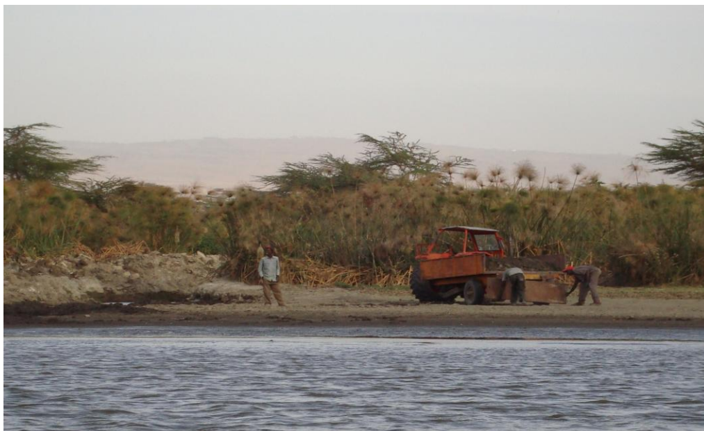
Plate 2-4: Motorised canal excavation works at the shoreline (Researcher 2009)
