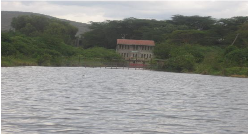
Plate 2-3: Oserian Pump House Lake Naivasha (Researcher 2009)
