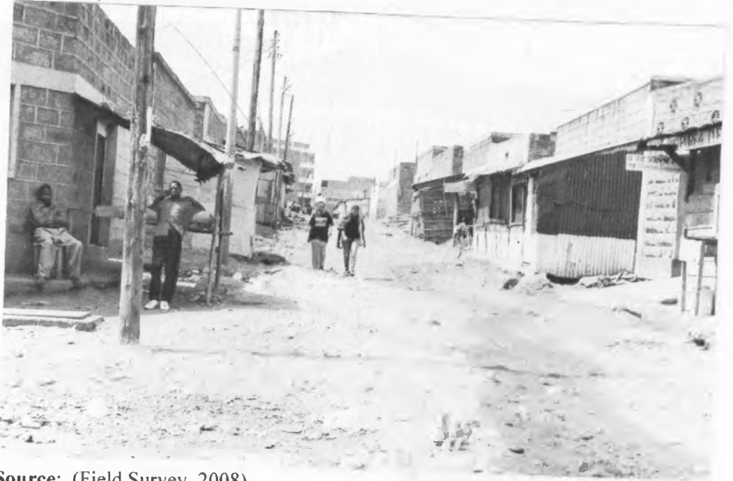
Plate 4.10 Access Road in Area 4 – Badly Worn Out (Note Encroachment on Road Reserve by Kiosks)
