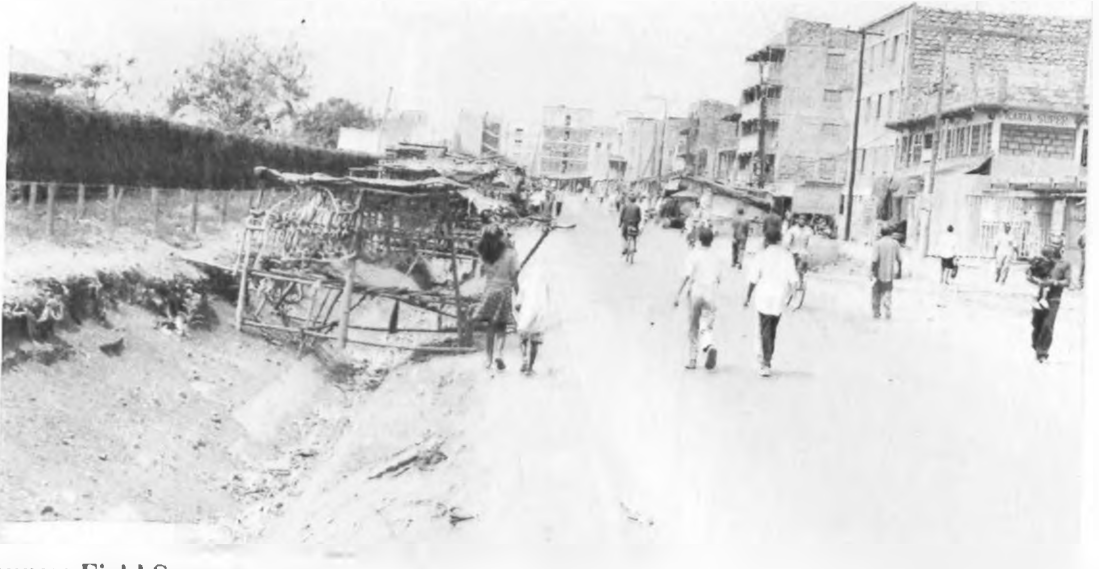
Plate 4.20: Structures Built Over Storm Water Drainage Along Northern Spin Road Making Cleaning of the Drain Difficult
