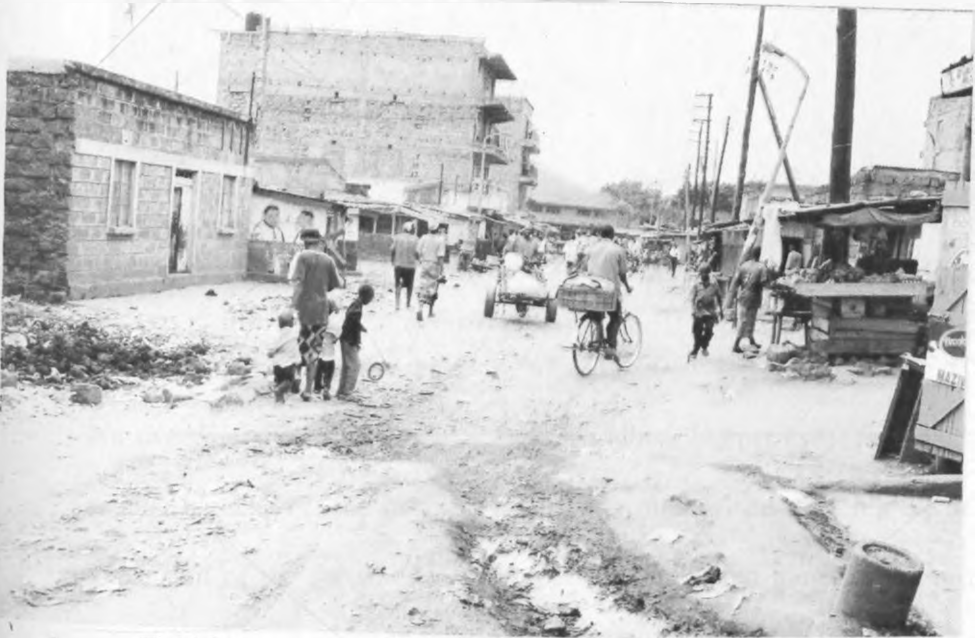
Plate 4.15 A Dilapidated Road in Area 4 (Note the depressions)
