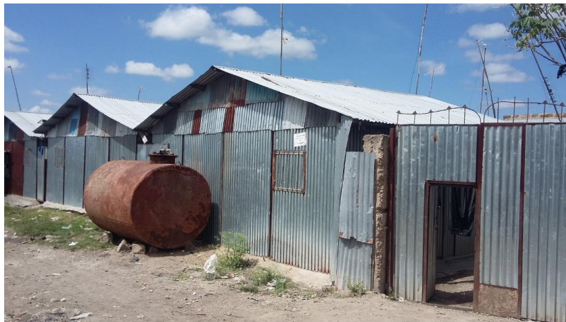
Plate 5-4: Connected Structures Source: Fieldwork, 2016
