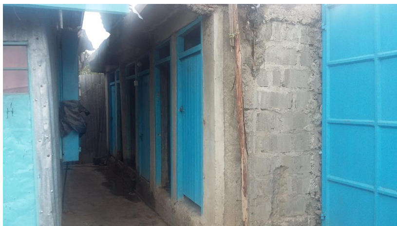
Plate 5-1: Washrooms within the Building Line Space
