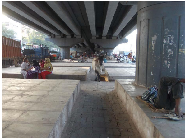
Plate 2. 9: The new platforms - not yet in use
