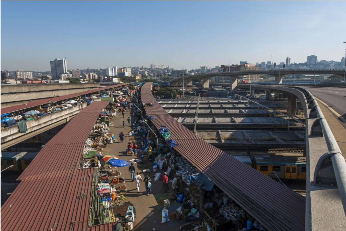
Plate 2. 16: Durban's Warwick Junction
