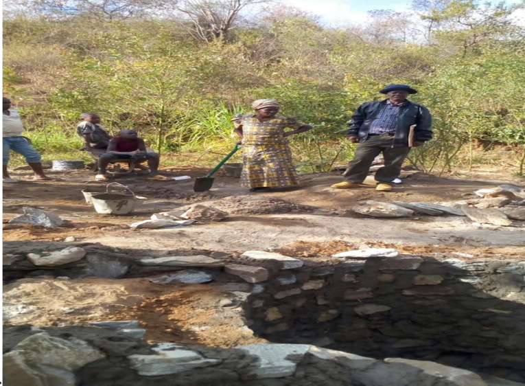
Plate 5. 2: Community members constructing a sand dam
