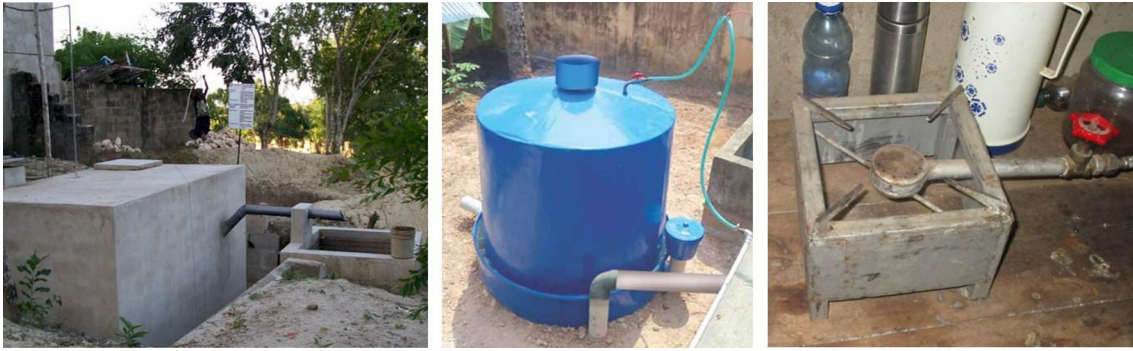
Photo 3. From left to right: VACVINA and plastic bio-digesters, biogas burner.
