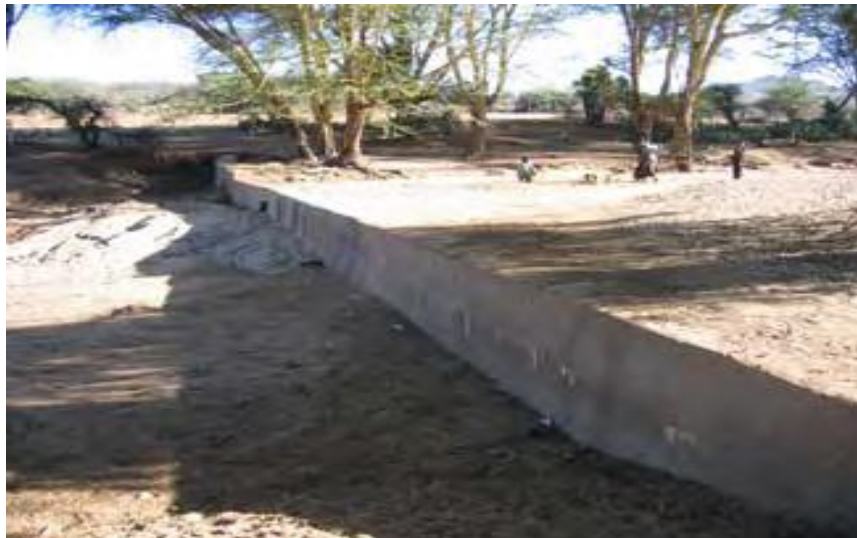
Figure 2: Sand Dam: Source AfDB RWH Manual 2008
