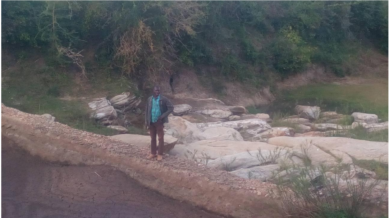
Figure 28: Stop Dam in Masii
