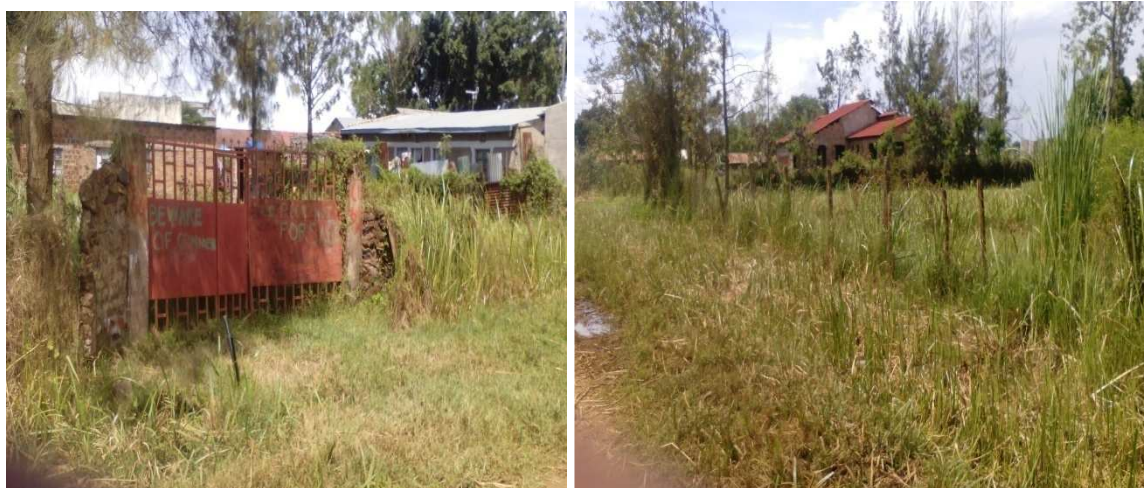
Fig 4.17: Construction right in the swamp
