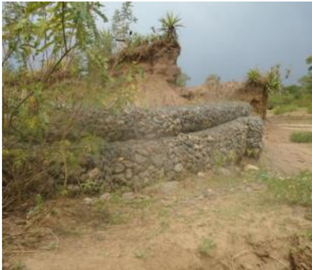
Figure 4.5: Gabions Constructed by Awach Kano WRUA Figure 4.6: Uncompleted Fish Pond
