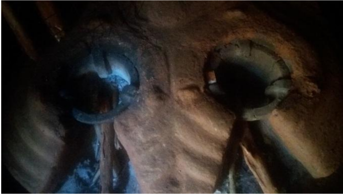
Plate 4.11 Fixed ICS observed in some households. Just 6 months old but have developed cracks and broken pot holder is observed.
