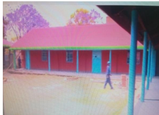
Fig: 4.8.3: Refurbished exterior
