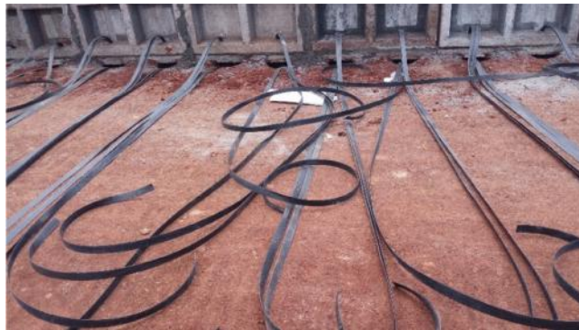
Plate 3-6: Sample geobelts erection on site
