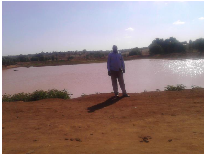
Plate 10: Kasovi earth dam
