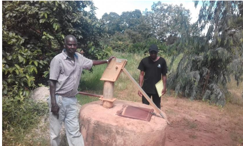
Plate 8: Shallow well equipped with a hand pump
