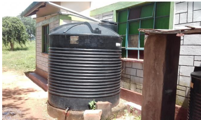
Plate 7: Household rooftop water harvesting (plastic tank)
