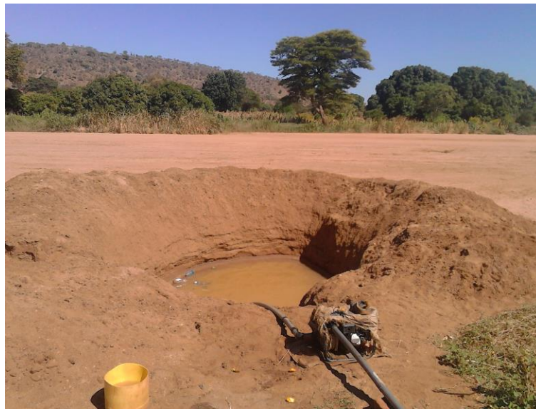
Plate 27: Shallow well dug at Dry tyaa river bed and used for irrigating vegetables
