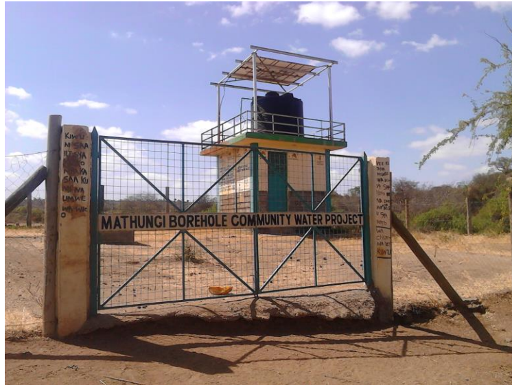
Plate 24: Mathungi Borehole Community Water Project
