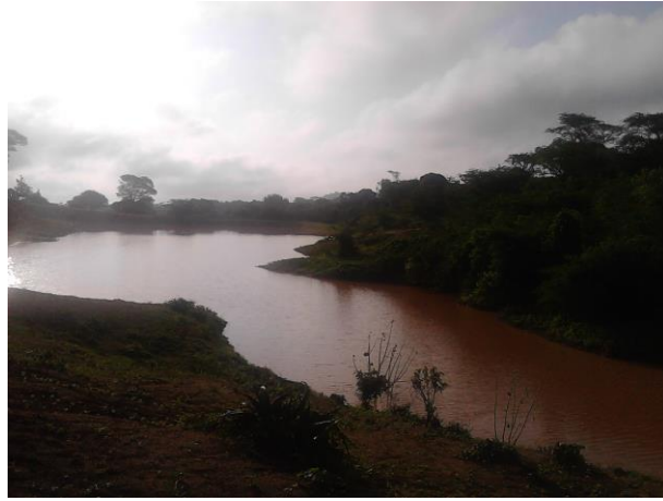
Plate 13: Kiia Earth Dam
