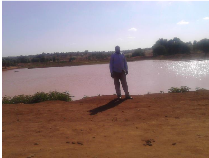
Plate 20: Kasovi Earth Dam
