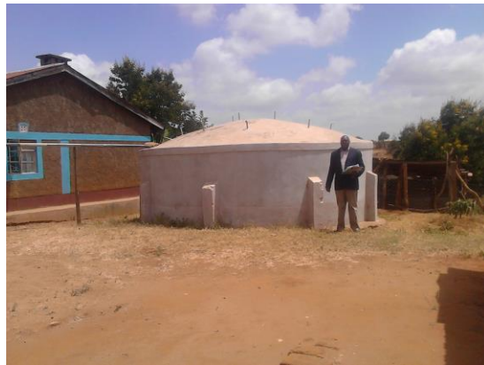
Plate 5: Household rooftop water harvesting (reinforced concrete tank)
