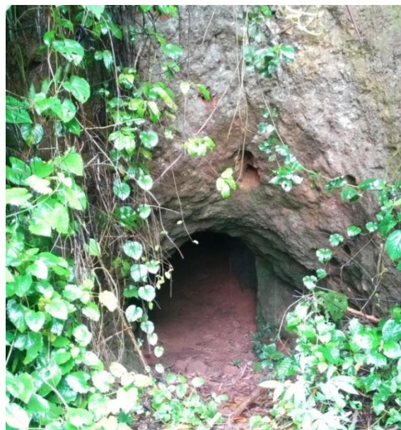
Figure 3-1: Main entry of the Bingo carbonatite adit at UTM coordinates X=758644; Y=62317
