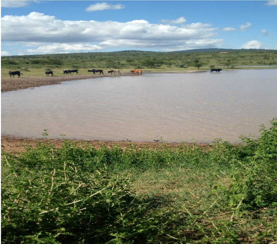
Figure 2: Dam in AMK with Animals Watering
