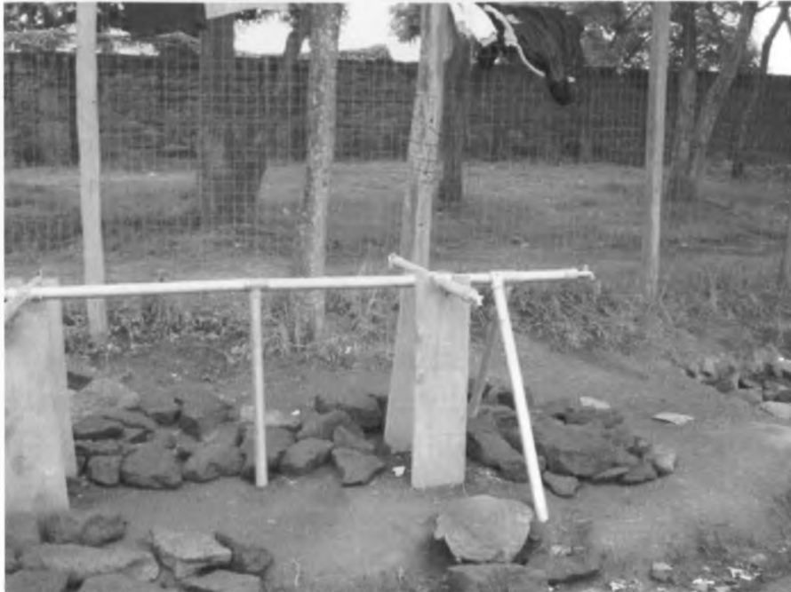
Figure 4: A piped water point at the camp
