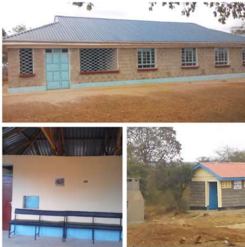
Image 4: The New Bosnia Dispensary in Makueni Sub County (Top: Main dispensary block, Bottom left: Waiting area, Bottom right: Medical waste disposal unit and pit latrine)
