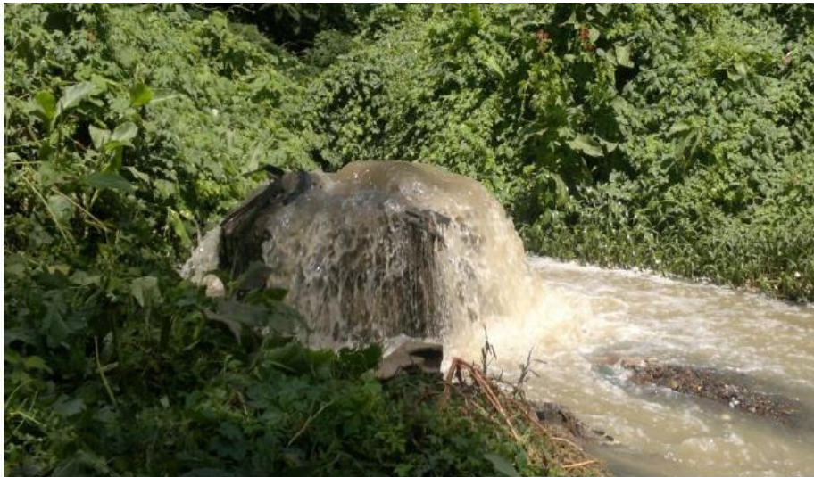
Plate 4: An open sewer flowing into Nairobi River at Michuki Memorial Park
