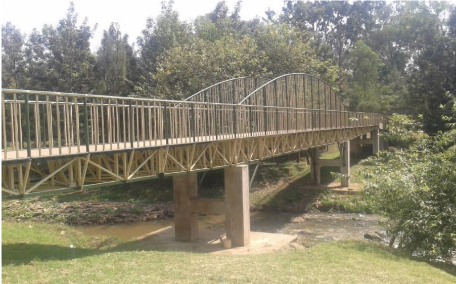
Plate 1: A section of the bridge connecting the two parts of MMP
