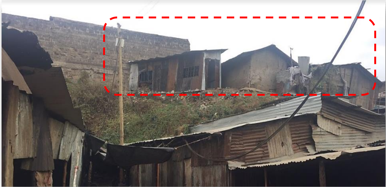
Figure 5.8: Houses on top of cliff at risk of landslides, with gradually eroding slopes
