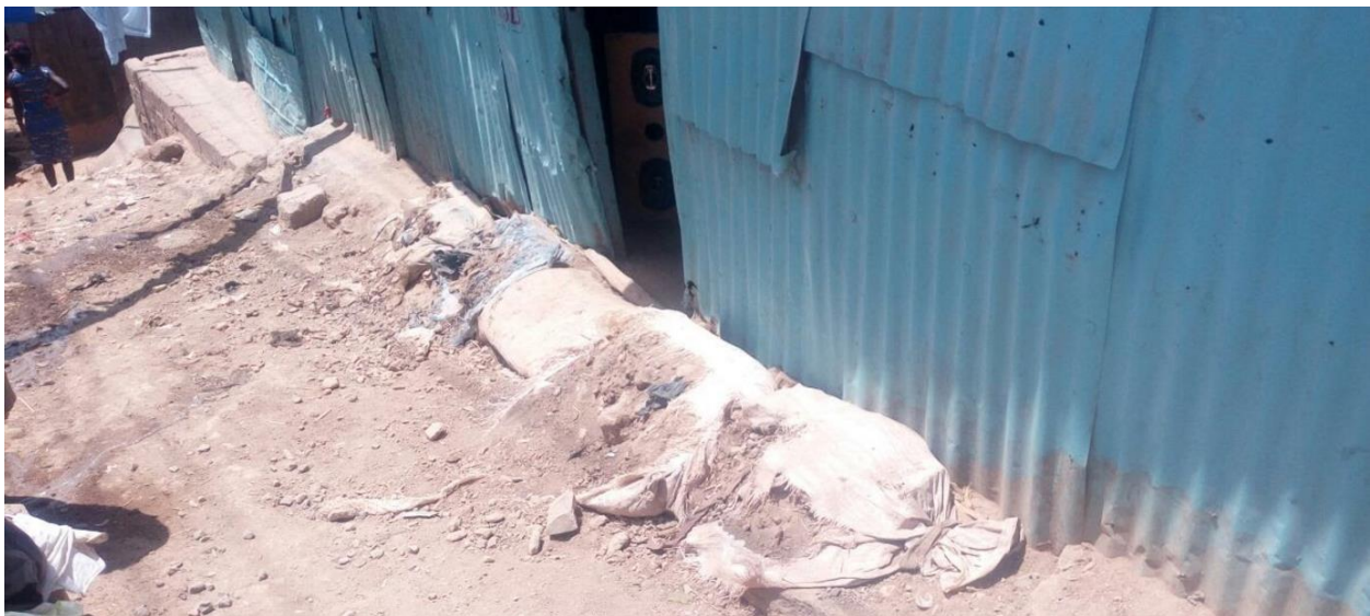
Figure 5.14: Sacks of sand laid at doorsteps to keep floodwaters out
