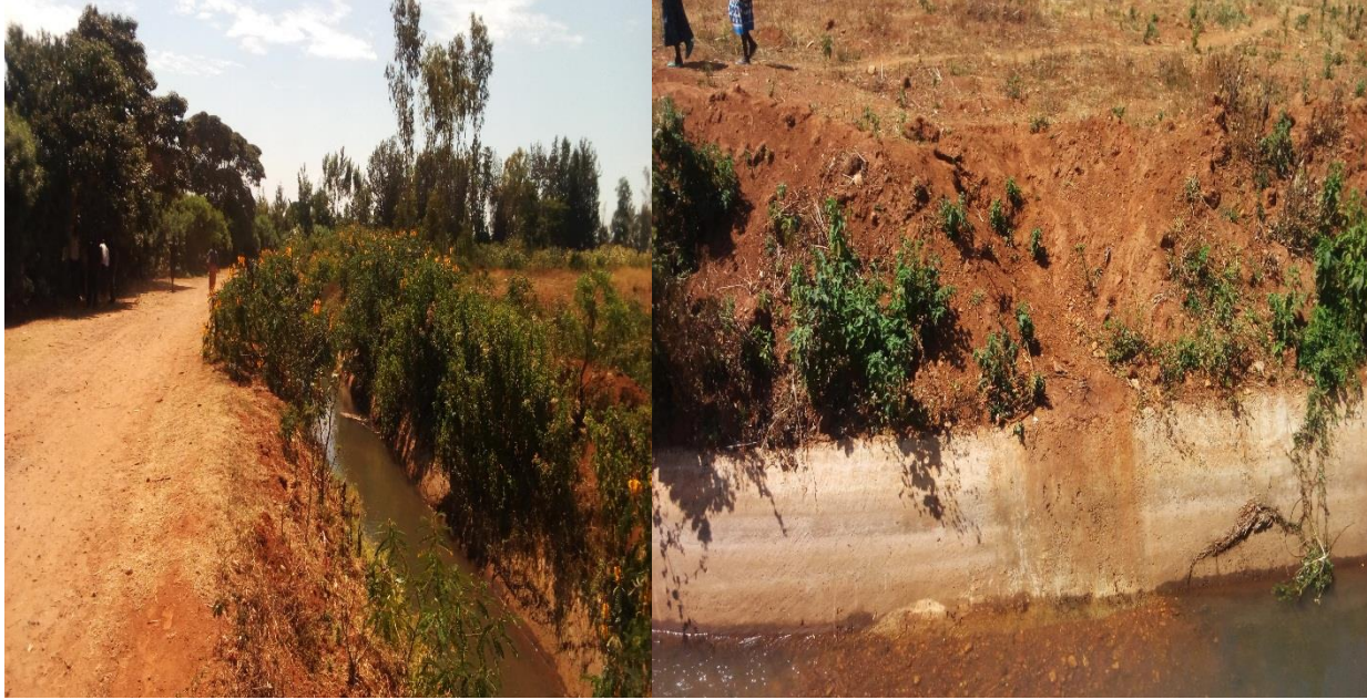
Figure 18: Siltation in the canal
