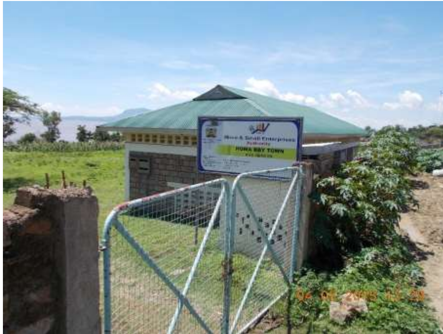
Picture 15: Homa Bay Town: The office of the MSE Authority.
