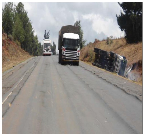
Plate 1.6: Rutting on Timboroa – Eldoret Road (Source: Kipyator F. K., 2013)
