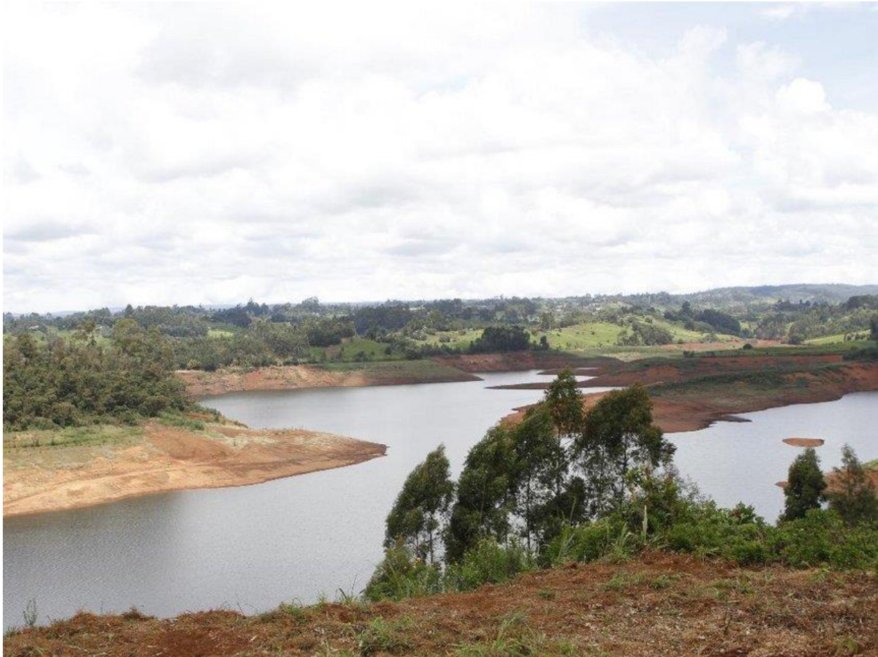
Plate 1.1: Ndaka-ini dam showing low water levels in rainy season April 18, 2018,
