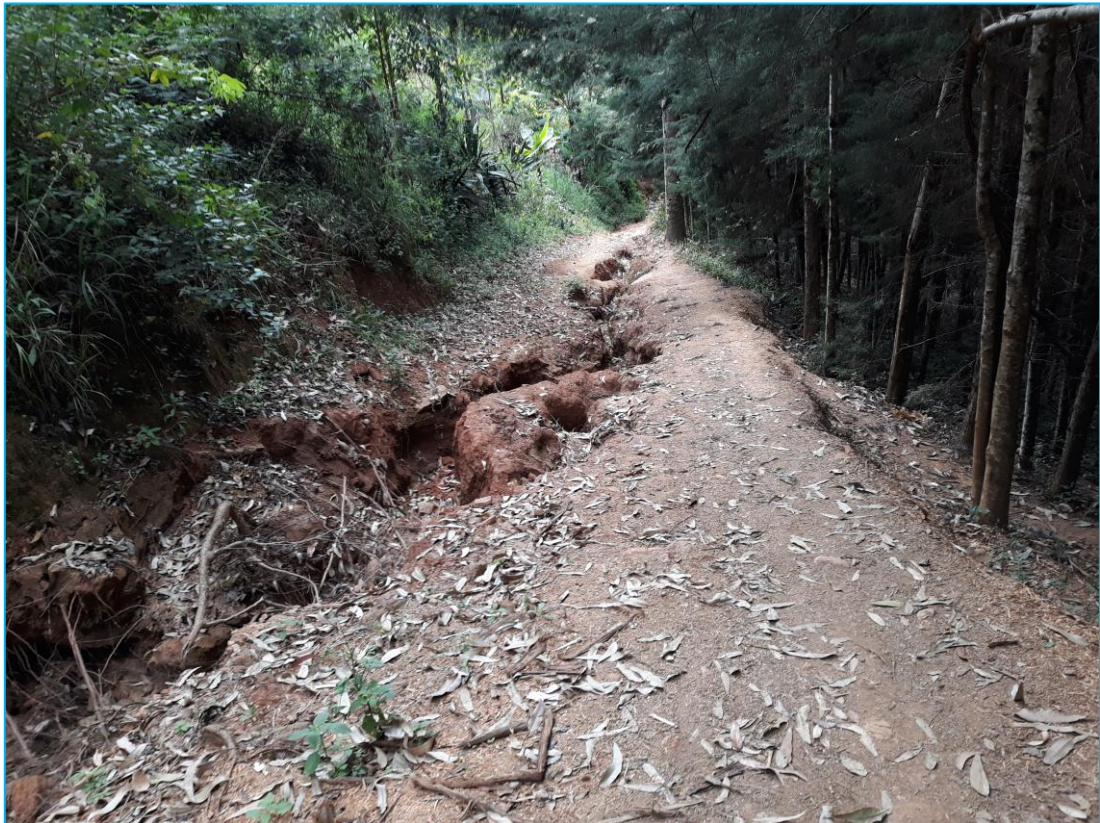
Plate 1: Poor State of an Access Road
