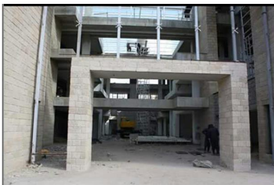
Figure 73: Construction of the entrance to the Strathmore Business School building.
