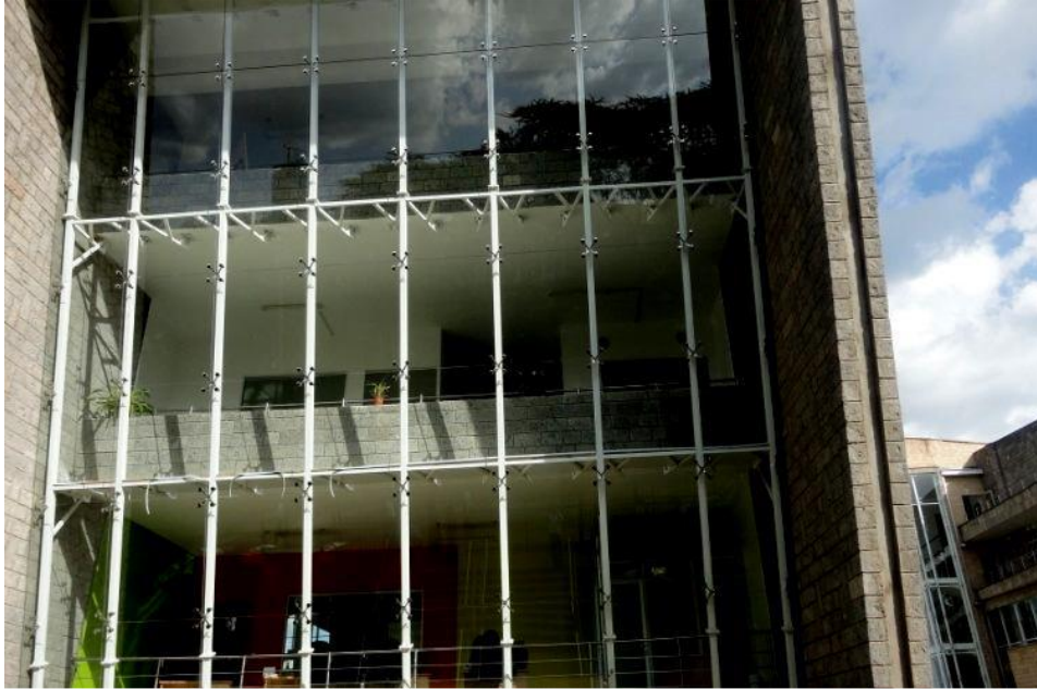
Figure 65: Glass curtain walls on the Strathmore Business School building. Source: (Strathmore Business School, 2012)
