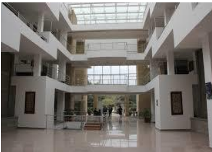
Figure 74: Internal finishes of the Strathmore Business School building. Source: Author, (Strathmore Business School, 2012)
