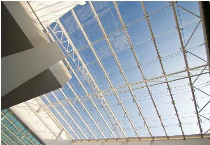
Figure 62: The atrium's glass roofing in the Strathmore Business School building.
