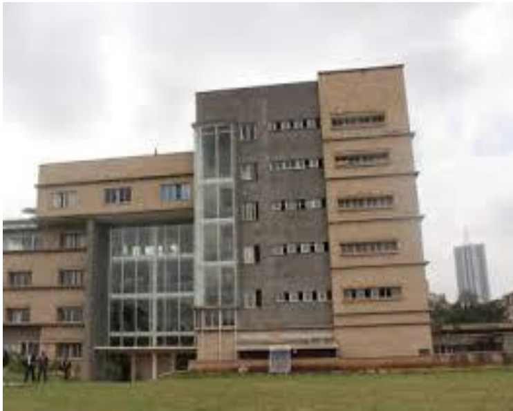
Figure 60: Openings on the Strathmore Business School building.
