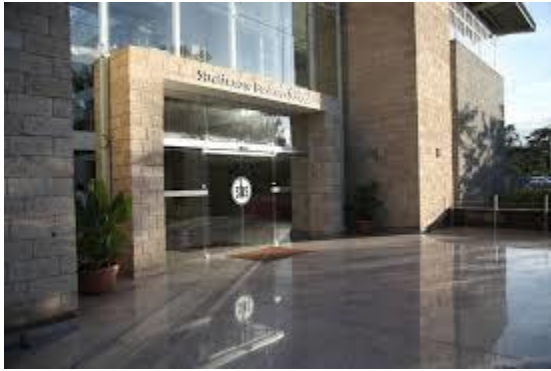
Figure 68: Strathmore Business School building's external finishes. Source: (Strathmore Business School, 2012)
