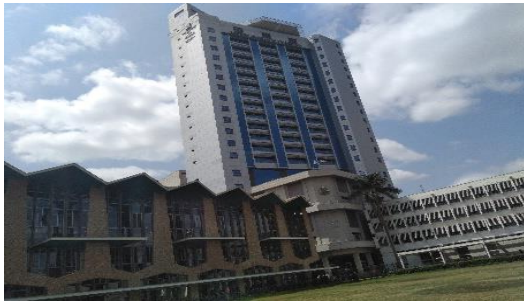
Figure 28: Existing buildings Source: Author, 2018
