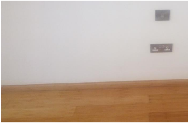
Figure 16: The smooth and light coloured finishes of the building
