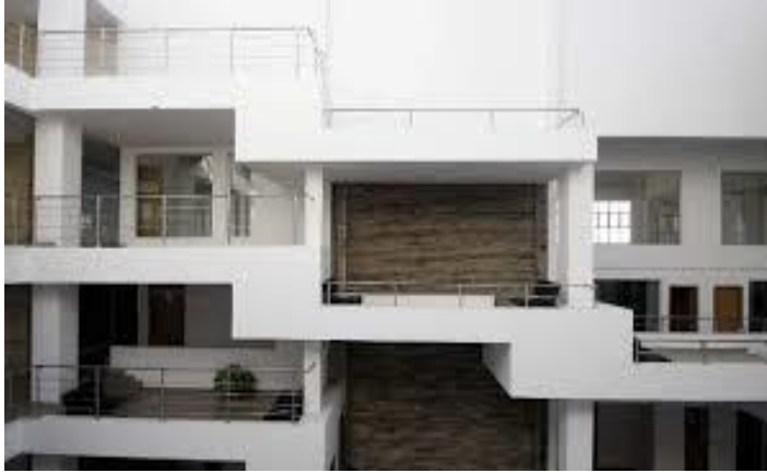
Figure 61: Strathmore Business School building's interior partitioning. Source: (Strathmore Business School, 2012)
