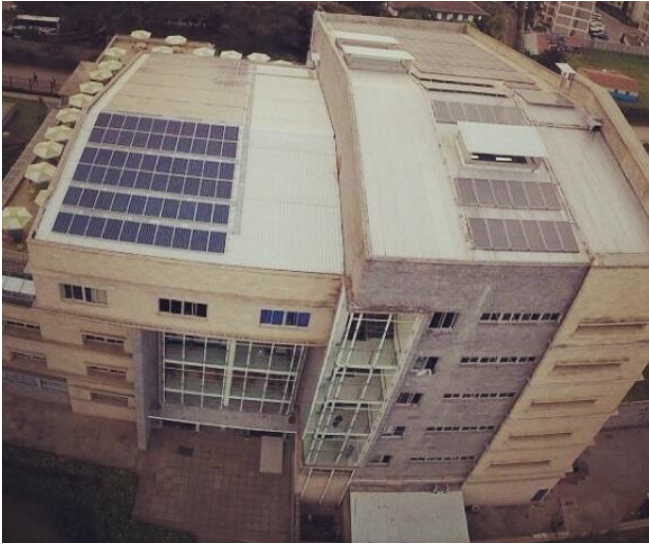
Figure 66: Strathmore Business School building's roof.
