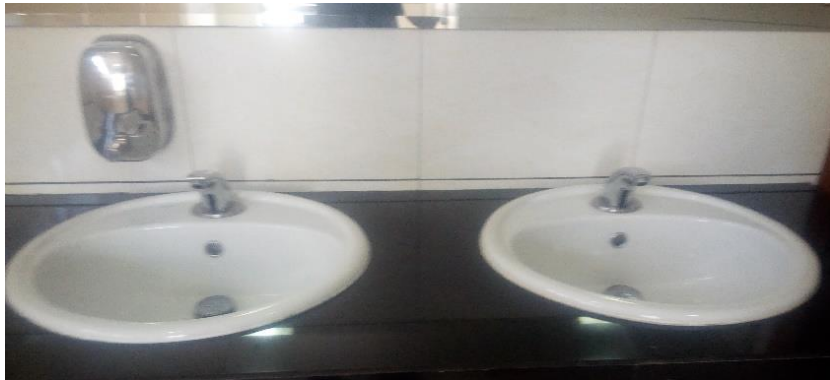
Figure 45: Water efficient taps used in the UON Towers Source: Author, 2018
