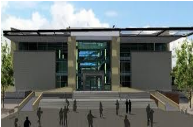
Figure 59: Strathmore Business School building - Form
