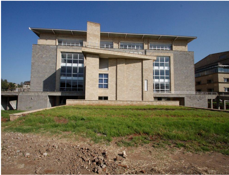
Figure 64: Roof overhangs on the Strathmore Business School building. Source: (Strathmore Business School, 2012)
