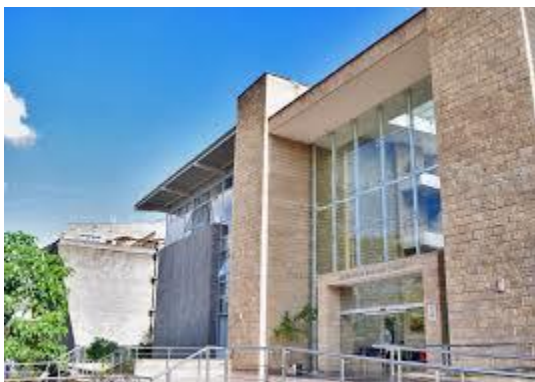
Figure 53: Strathmore Business School building's exterior.
