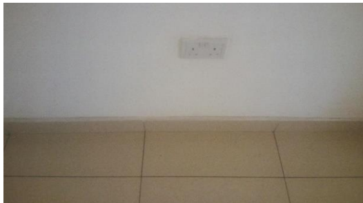
Figure 41: Finishing of the building
