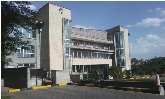
Figure 52: Car parking spaces outside the Strathmore Business School building Source: Author
