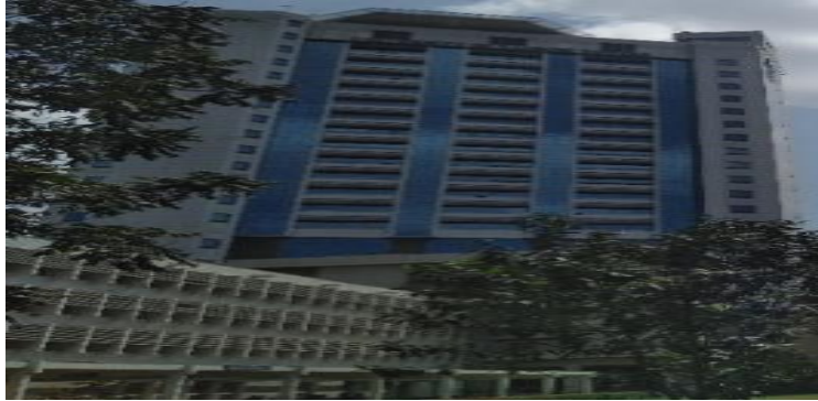
Figure 39: Glazed windows of the UON Towers
