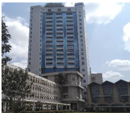
Figure 20: Windows in the University of Nairobi Towers. Source: Author, 2018
