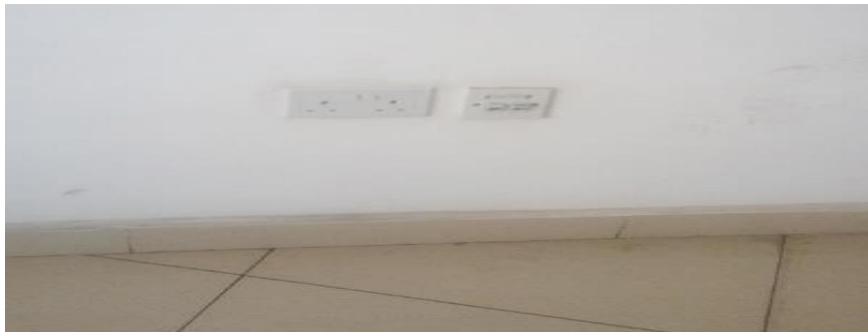
Figure 44: Internal texture of the UON Towers
