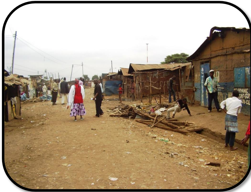
PLATE IV: ROAD C, BEFORE UPGRADING
