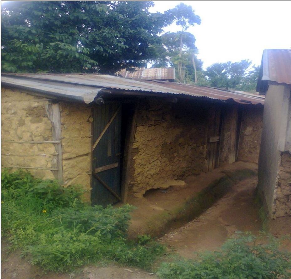
Plate 1: House with Wall Made of Mud
