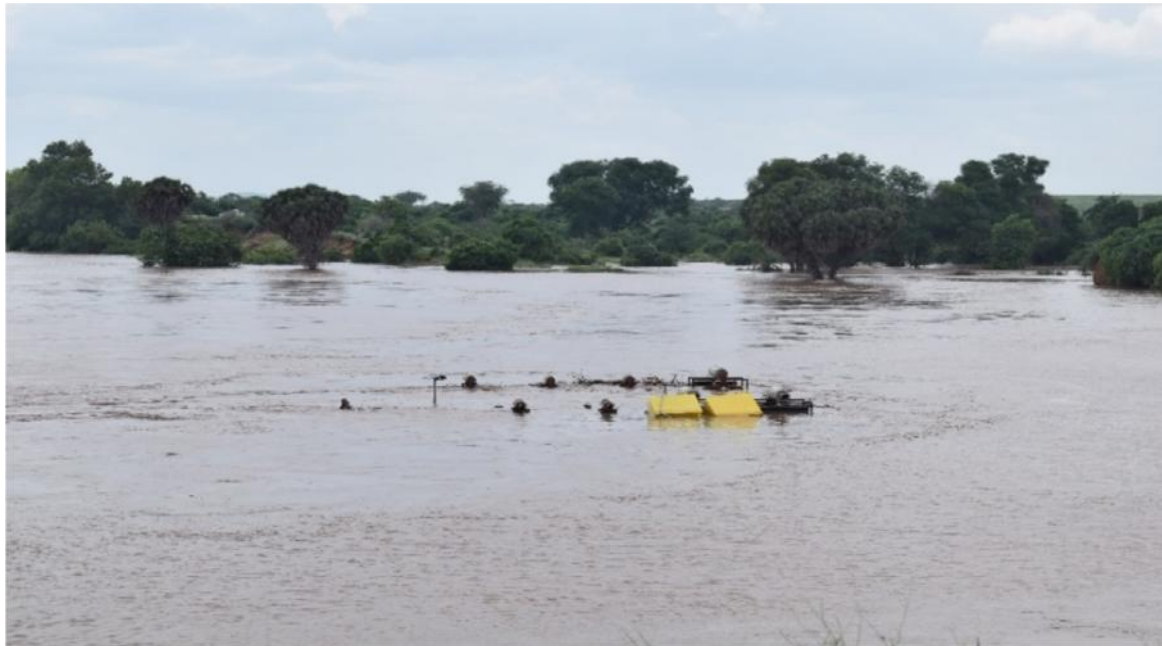
Figure 4: Effects of floods on the project in May 2018
