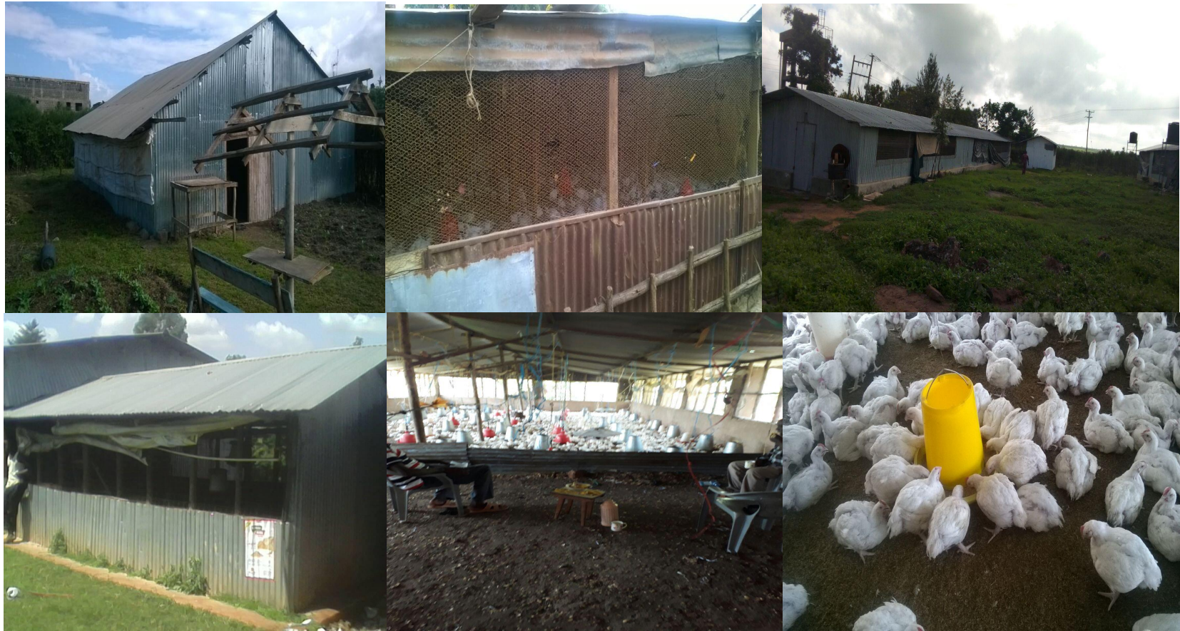
Figure 4.3: Broiler chicken housing showing different types of materials used for construction of walls and roofs and litter
